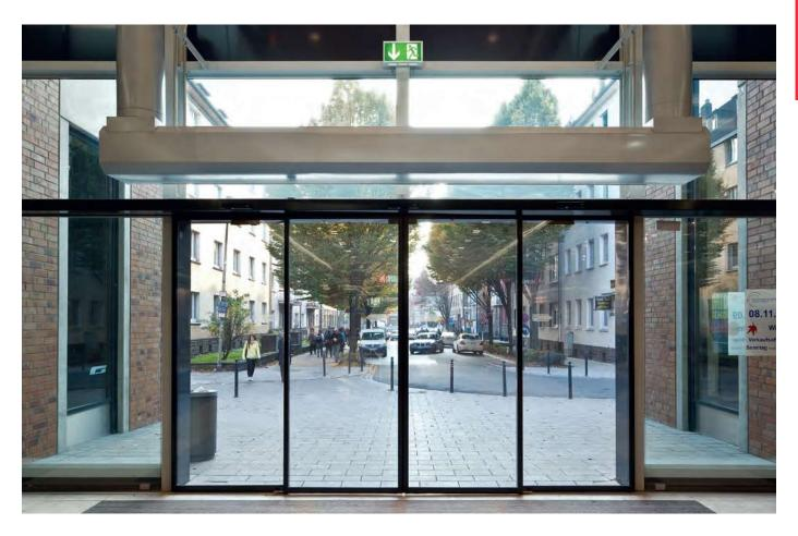
Swing-out door leaves and side panels can open up very large passageways in the event of danger. In automatic mode, the breakout sliding door functions like a standard sliding door.
